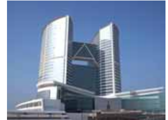
JAFZA Convention Centre, Office, & Hotel Bldg
