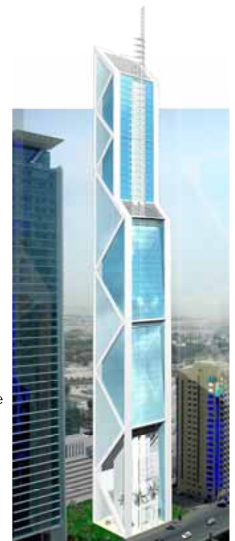
G+62 Hotel in Shk Zayed Rd.
